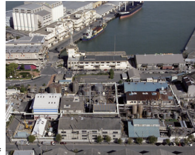
Panoramic View of Yokkaichi Branch
