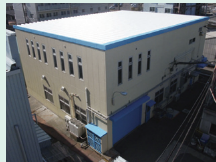
Cafeteria building coated with heat insulation paint
