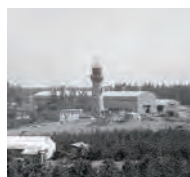
Builds the Ohgata Plant, the first facility in Japan to commence manufacturing of solvent-method CMC (CELLOGEN)
