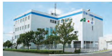
Kasumi Plant (Yokkaichi City)
