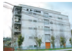
1970 Constructs sucrose fatty acid ester plant
